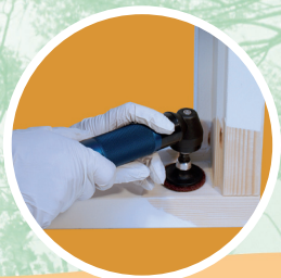
1. Remove paint & dirt
