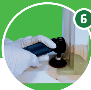
Sand finished repair
