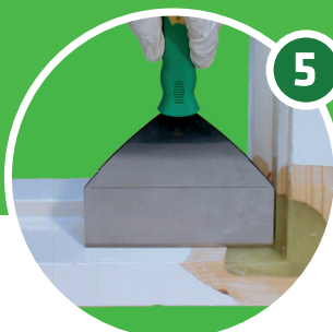
Shape and finish repair
