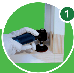
Remove paint & dirt
