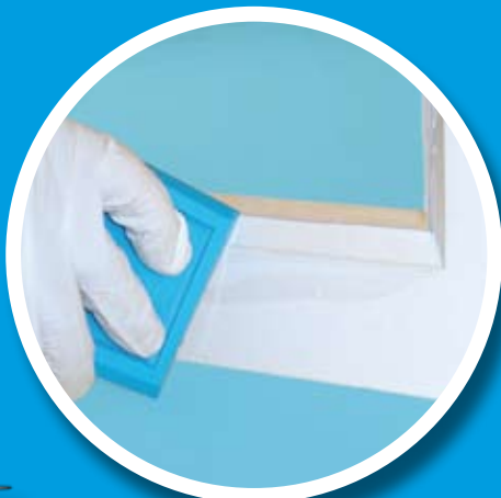
6. Smooth the surface by holding the applicator up-right
