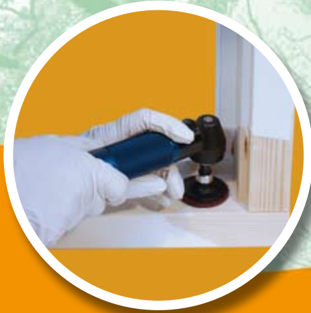
1. Remove paint & dirt
