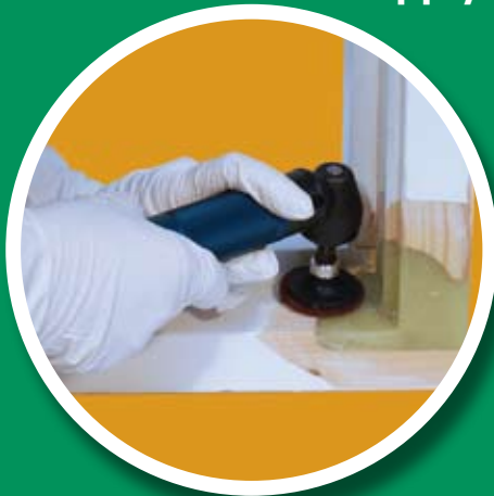
6. Sand finished repair
